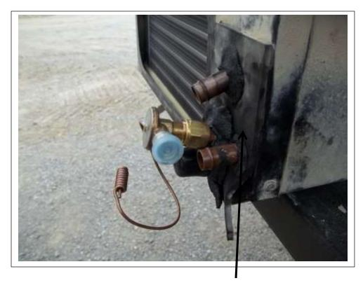
Seal all openings around the tubes with tar tape as shown.
