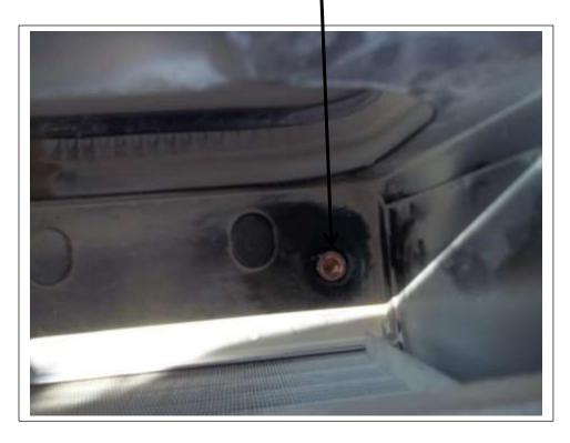
Install the short drain tube onto the copper extension previously glued into the box on the fitting end of the box. Add the drain tube restrictor and tighten the clamps.
