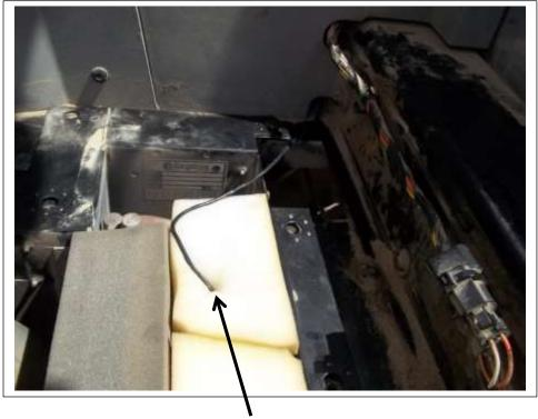
Insert about 6" of the thermostat probe into the evaporator coil as shown between the second and third rows of the coil. Note this area will already have the 1/8" foam on it. Install the probe through it as well.
